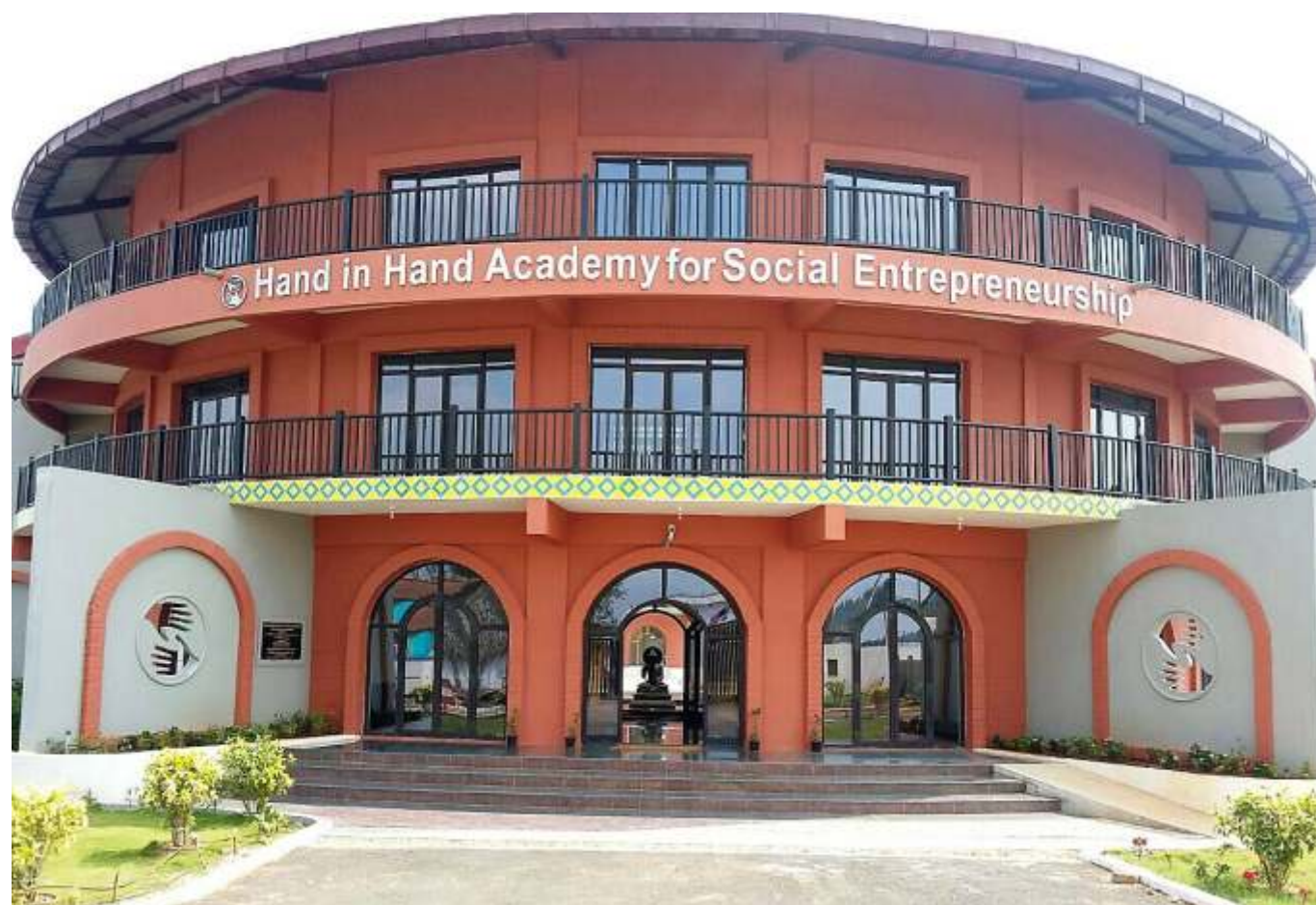
A photograph of the front façade of the training building showing the client's logo integrated into the building design along with the custom tiles made using the client's greeting card design.
