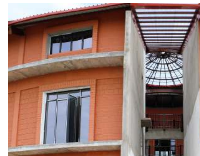
The unplastered exterior wall constructed from hollow terracotta blocks.
