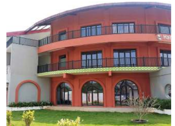
A photograph of the large, well shaded windows fitted with solar control glass
