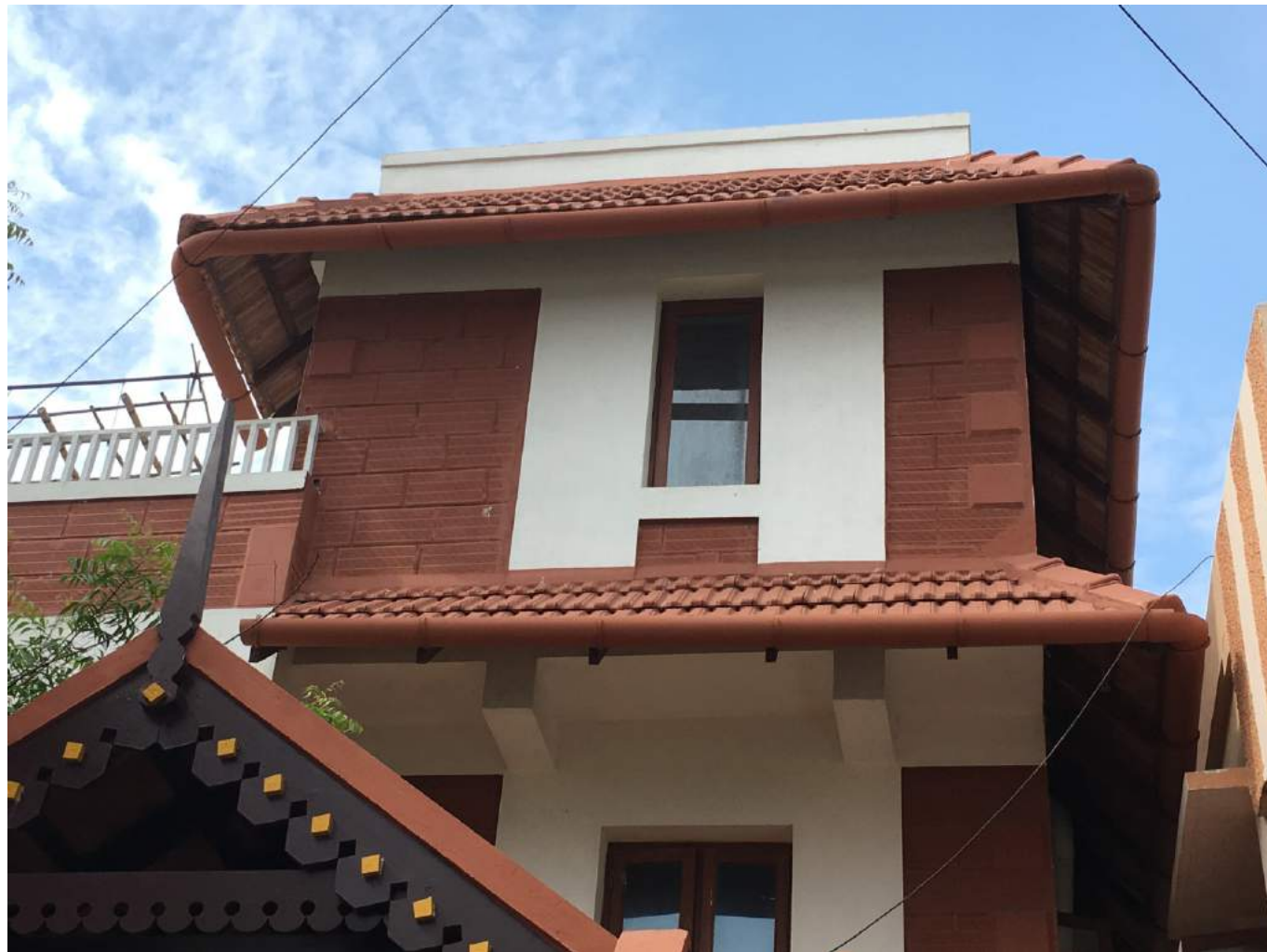
Insulating hollow terracotta blocks, well shaded windows with solar control glass
